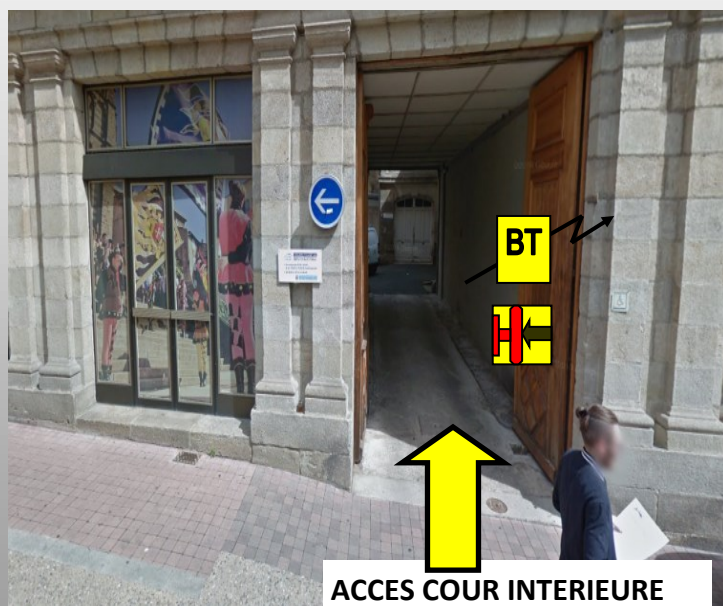
FACADE PLACE DU PLOT
